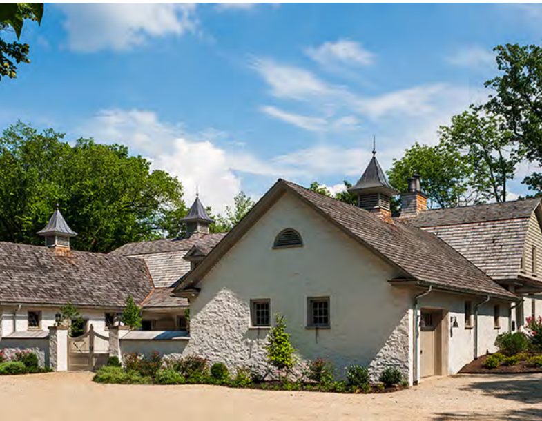
~ E.C. Trethewey Building Contractors ~ Downingtown ECTBuilders.com
