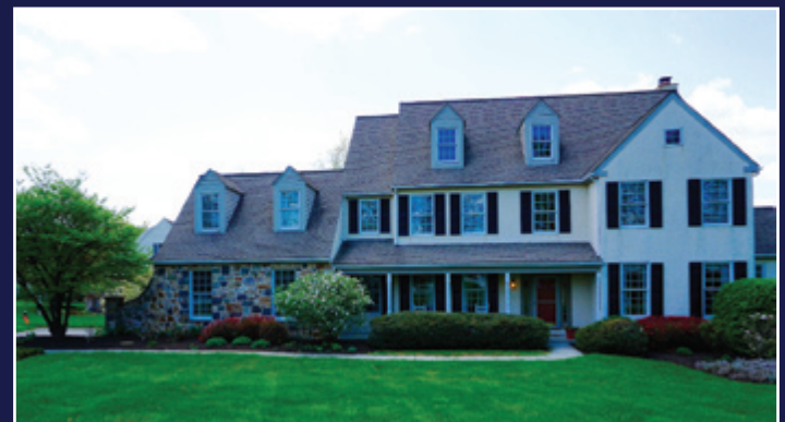
Saint Peters Way | W. Pikeland Township | .33 Acres Gourmet Kitchen with Breakfast Room | Great View off Trex Deck
